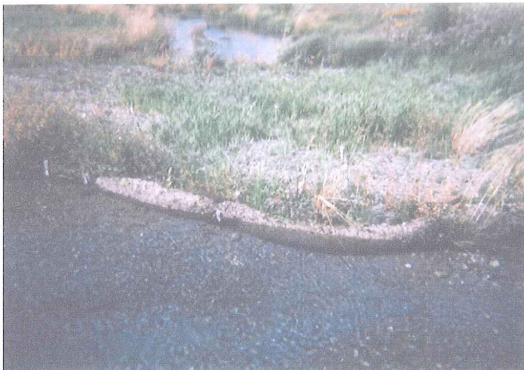
Illustration 2. Restoration efforts on Upper Grove Creek, occurred in 2002 and 2004 with the use of Biologs to narrow stream channels.
