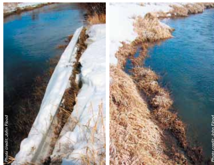
Overhanging bank collapses in Silver Creek during winter conditions
