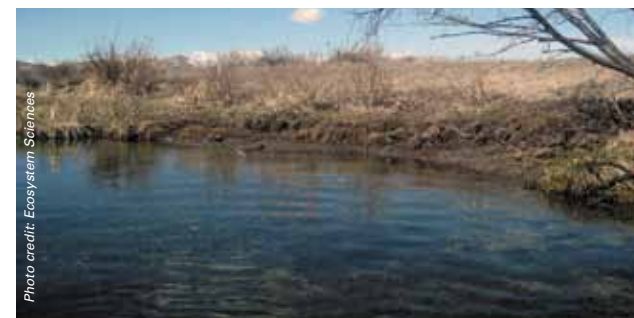
Bank erosion on Silver Creek
