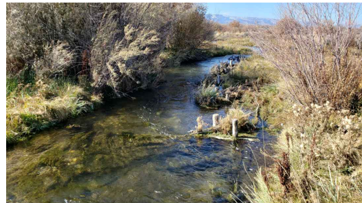
ABOVE: 1-YEAR POST-CONSTRUCTION; SMALL WOODY DEBRIS STRUCTURES (BIG SPRINGS CREEK, ID)
