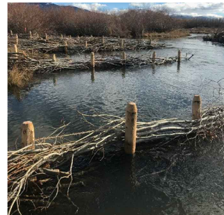
ABOVE: POST LINE WILLOW WEAVE CONSTRUCTION (LEMHI RIVER, ID)
