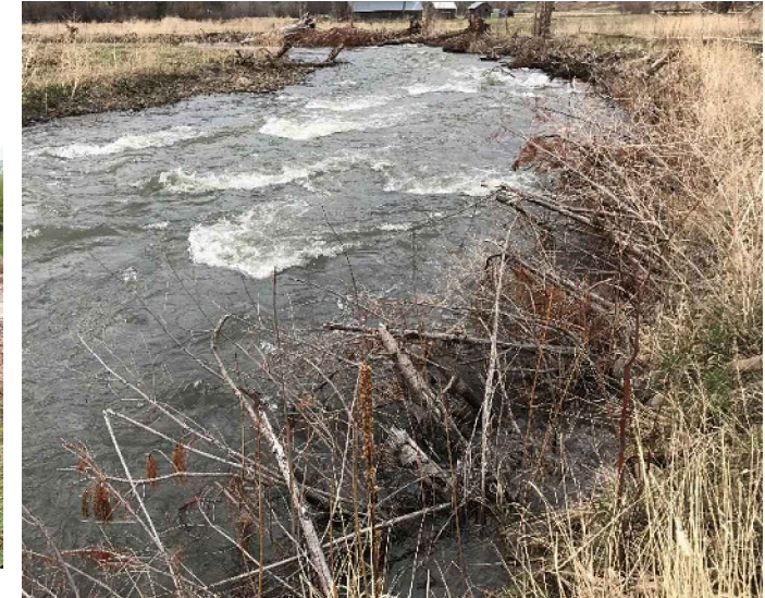
BELOW: SLASH BRUSHLAYER 1-YEAR POST CONSTRUCTION (CATHERINE CREEK, OR)
