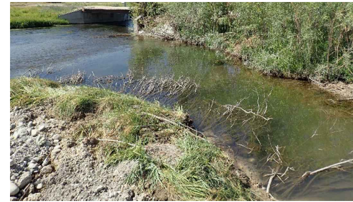
ABOVE: WILLOW BRUSHLAYER IMMEDIATELY AFTER CONSTRUCTION (LEMHI RIVER, ID).
