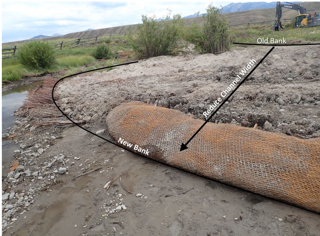
Figure 4-12. Bank Fill Treatment Example
