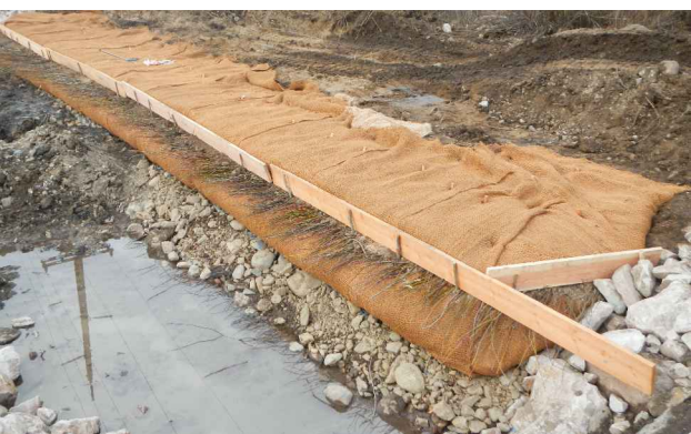
ABOVE: FESL CONSTRUCTION WITH LIVE WILLOW BRUSHLAYER (YANKEE FORK, ID).
