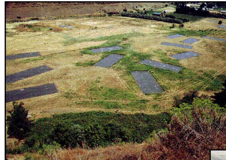
ABOVE: RIPARIAN PLANTING STRIPS DURING CONSTRUCTION IN YEAR 2001 (WALLA WALLA RIVER, OR)
