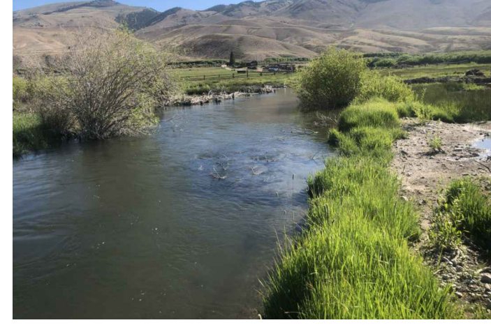
BELOW: BANK FILL WITH WETLAND SOD BANK 1-YEAR POST-CONSTRUCTION (LEMHI RIVER, ID)
