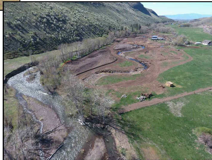
BELOW: CHANNEL RE-MEANDER/RECONSTRUCTION OCCURRING WITHIN FLOODPLAIN (CATHERINE CREEK, OR)
