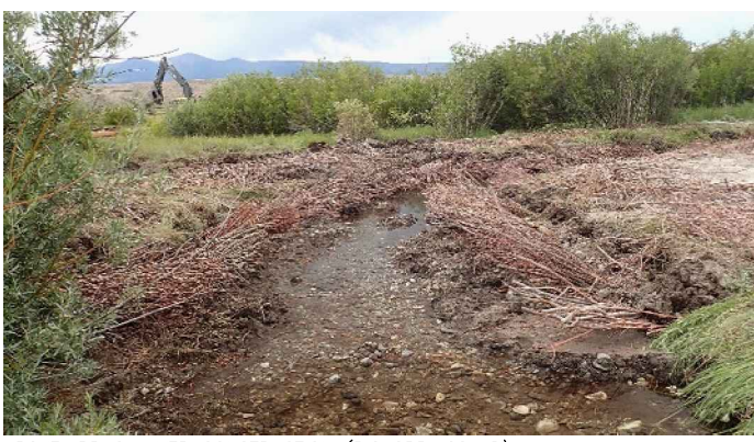
ABOVE: BRUSHLAYER CONSTRUCTION (BIG SPRINGS, ID).
