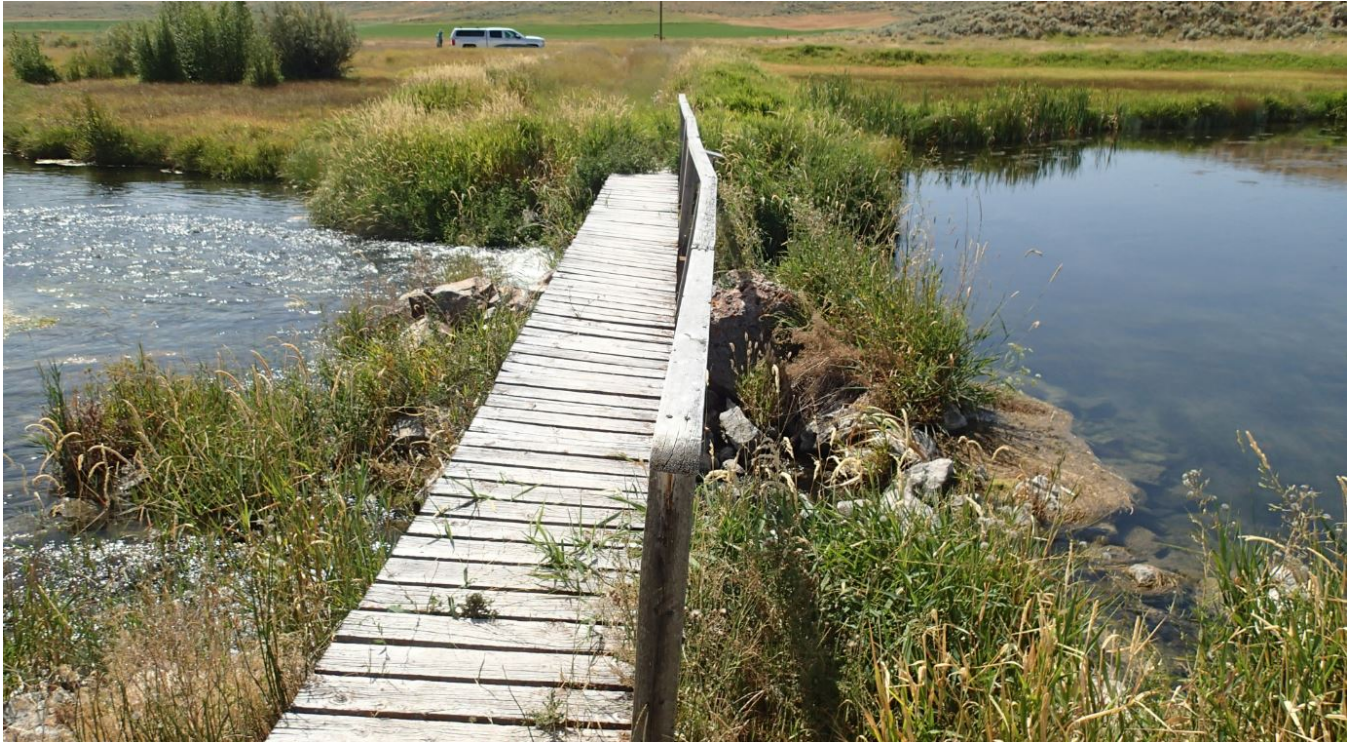
Figure 6-5. Rock Check Dam in Lower Stalker Creek
