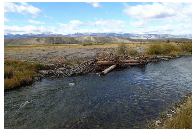
ABOVE: IMMEDIATELY POST-CONSTRUCTION; LARGE WOODY DEBRIS HABITAT STRUCTURE (LEMHI RIVER, ID)
