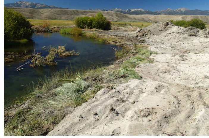
ABOVE: WETLAND SOD BANK IMMEDIATELY POST-CONSTRUCTION (BIG SPRINGS CREEK, ID).
