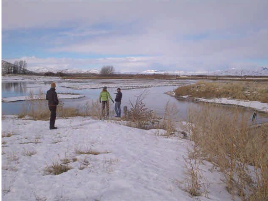
Plate 1. View upstream of Kilpatrick Pond from Purdy dam. Dam structure is on right edge of photo.
